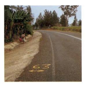
Fig 4.25 Road in Papua New Guinea with shallow side slopes and rounded drainage ditches improves safety (TRL)
