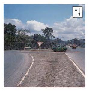
Fig 4.74 Roundabout in Papua New Guinea with insufficient deflection permitting vehicles to pass though without reducing speed, e.g. yellow vehicle (TRL)
