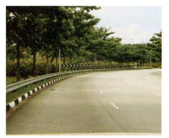
Fig 6.25 Well defined curve in Singapore, guiding drivers and giving ample information of road geometry ahead (TRL)
