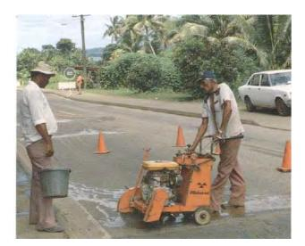
Fig 5.12 Cutting out damaged road surface with diamond saw, Fiji (Ross Silcock Partnership)
