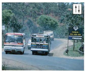
Fig 6.27 Dangerous overtaking on a steep winding road in Indonesia with many HGVs and buses but no crawler lanes (TRL)
