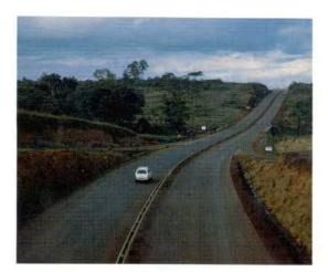
Fig 6.36 Median barrier on rural road in Kenya prevents U-turns and crossover accidents (Rendel Palmer & Tritton)
