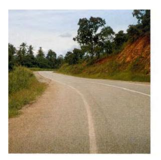
Fig 4.12 Superelevation on road in Papua New Guinea (TRL)
