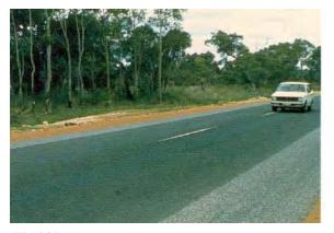
Fig 4.37 Shoulder delineation by use of different coloured surfacing in Australia (Rendel Palmer & Tritton)
