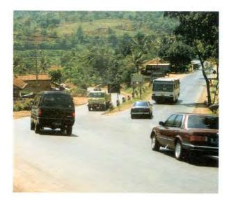
Fig 4.71 Poorly designed T-junction in Indonesia with no road markings and very poor sight-Line in one direction (TRL)
