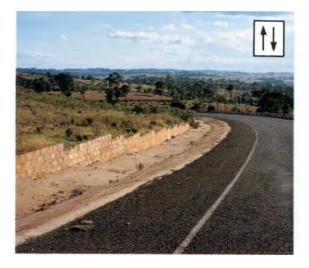
Fig 4.28 Shallow slope to drainage channel gives room for recovery in Kenya
