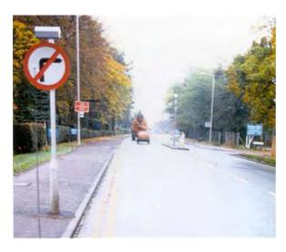
Fig 6.51 Banned right turn in UK. Note small channelising island to prevent turning manoeuvre at T-junction (TRL)
