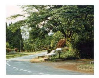
Fig 4.81 Dangerous T-Junction in Zimbabwe due to very poor sight lines (Zimbabwe Traffic Safety Board)
