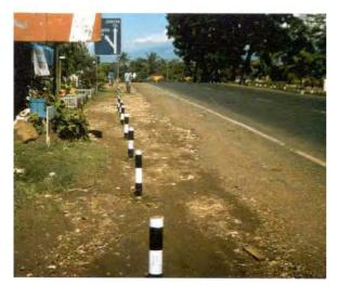
Fig 6.39 Edge lines and painted bamboo posts provide low cost delineation in Indonesia (TRL)
