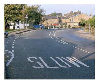
Fig 6.22 Improvement to intersection shown in Fig 6.20 to increase conspicuity and give emerging drivers a better view (TRL)
