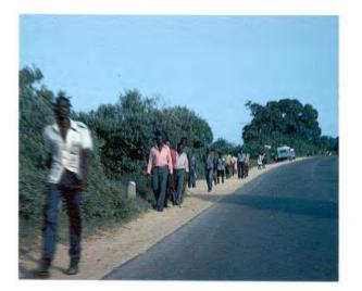
Fig 4.58 Narrow shoulder on paved rural road in Africa provides some protection but inadequate for volume of usage (Ross Silcock Partnership)
