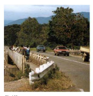
Fig 4.33 Guard rail to protect pedestrians on bridge, Papua New Guinea. Note flared barrier end treatment to minimise consequence of impact (TRL)
