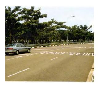
Fig 6.40 Curve delineated by painted kerbs and chevrons. Note also crash barrier and speed reduction markings, Singapore (TRL)
