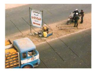
Fig 5.04 Axle detectors linked to roadside equipment in Egypt to monitor flow and enforce speed limit (TRL)
