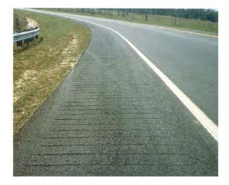
Fig 6.26 Rumble strips on shoulder to alert drivers who have strayed from carriageway before bend ahead, USA (Ministry of Construction. Korea)
