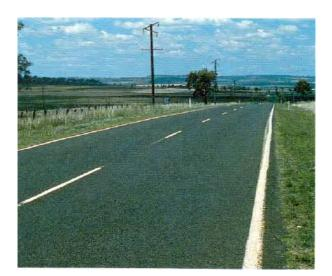
Fig 6.31 Clearly defined centre line and edge line, Australia (Rendel Palmer & Tritton)
