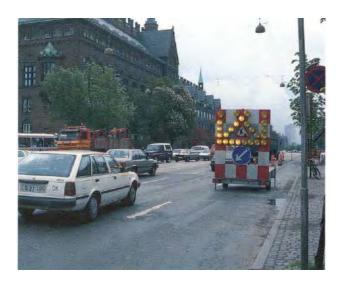
Fig 5.11 Illuminated temporary sign used to give clear warning of roadworks to drivers, Denmark (TRL)
