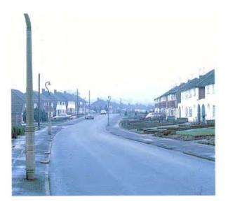
Fig 3.24 Long, straight and wide local distributor encouraging high speeds in the UK (TRL)
