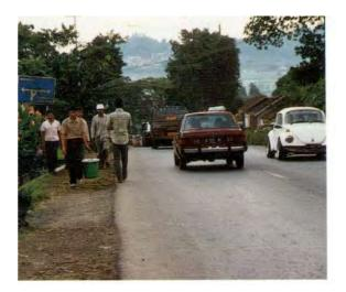
Fig 3.23 No pedestrian facilities on this local distributor in Indonesia (TRL
