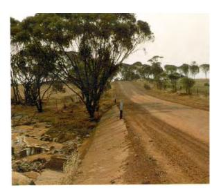
Fig 6.37 Inadequate edge delineation with steep ditch and roadside trees in Australia (Rendel Palmer & Tritton)
