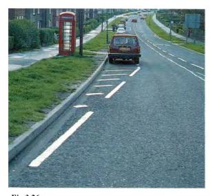
Fig 3.26 Local distributor in the UK where carriageway has been narrowed by protected parking to reduce speeds. Note well separated footway (TRL)
