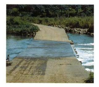
Fig 4.84 Unmarked ford - absence of advance warning creates potential danger. Note scour on downstream side (Rendel Palmer & Tritton)
