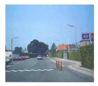
Fig 5.37 30 km/h speed limit in a special residential area in Denmark. Note speed humps (Ross Silcock Partnership)
