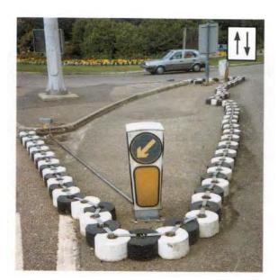
Fig 4.76 Experimental alteration to prevent overtaking on exit from roundabout and provide larger refuge for pedestrians (TRL)
