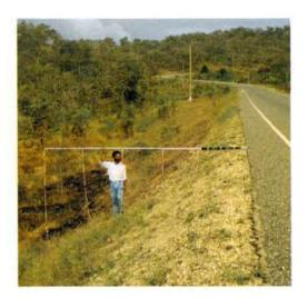
Fig 4.23 Severe unprotected side slopes being surveyed in Papua New Guinea (TRL)
