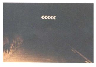
Fig 5.26 Reflectorised Chevron warning sign in Papua New Guinea is readily visible at night (TRL)
