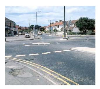
Fig 6.18 Double mini roundabout used in the UK for staggered cross roads (TRL)
