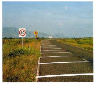
Fig 4.09 The substandard bend of Fig 4.07 after low-cost treatment of chevron board and bar line road markings (TRL)
