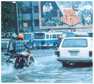
Fig 5.05 Poor drainage and inadequate maintenance leads to flooding of carriageways in Thailand (JMP Consultants Ltd)
