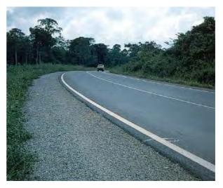
Fig 6.24 Incorrect superelevation and inadequate signing has resulted in a high accident rate on approach to bend in Ghana (TRL)
