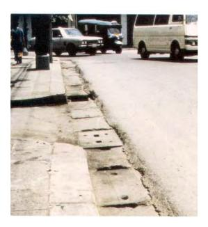
Fig 4.29 Covering drainage channels as In Thailand can reduce the risk of accidents such as shown in Fig 4.27 (JMP Consultants Ltd)
