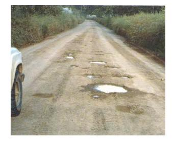
Fig 5.10 Poorly maintained road in Papua New Guinea, damages vehicles and presents danger to traffic (Rendel Palmer &. Tritton)
