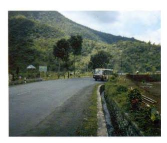
Fig 4.05 Poor sight distance on a curve in Indonesia. Note also Utype drain which poses potential hazard (TRL)
