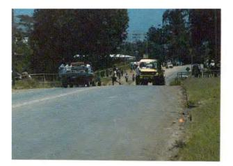
Fig 4.13 Poor visibility due to sag curve in Papua New Guinea (TRL)
