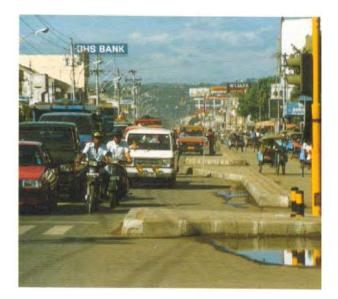
Fig 5.39 Poorly designed protected parking bays in Indonesiacollisions occur with kerbs particulary at night (TRL)
