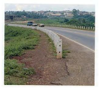
Fig 3.22 Vehicle barrier in Ghana prevents direct access and provides protected footway. However, note unsafe, exposed end post (TRL)
