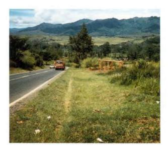
Fig 4.41 Vegetation and shelter well clear of roadside in Papua New Guinea, reduces risk of collision (TRL)
