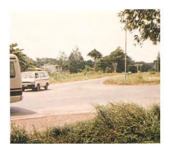
Fig 5.27 Inadequately marked T-Junction in Papua New Guinea offers little guidance to drivers (TRL)
