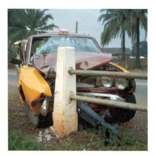
Fig 4.31 Vehicle impaled on incorrectly terminated barrier, Ghana (TRL)
